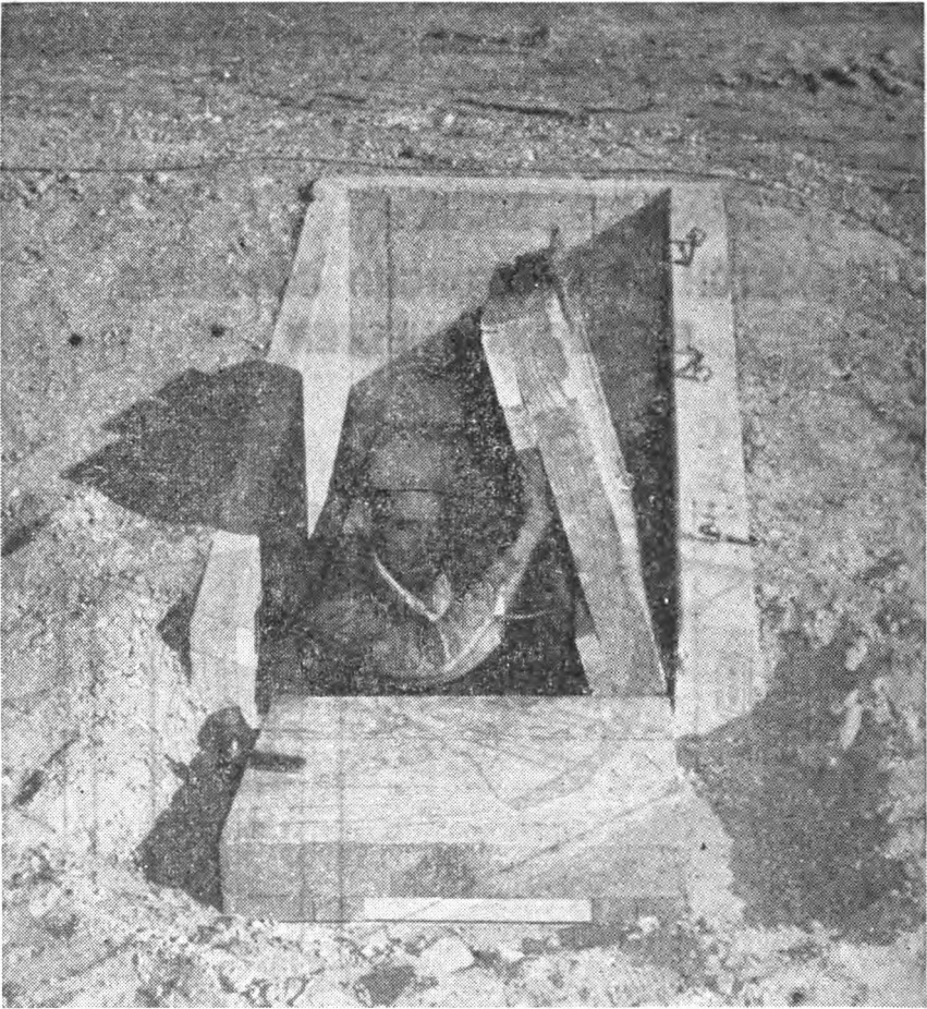
SLIDE No. 11.—Family underground shelter.
